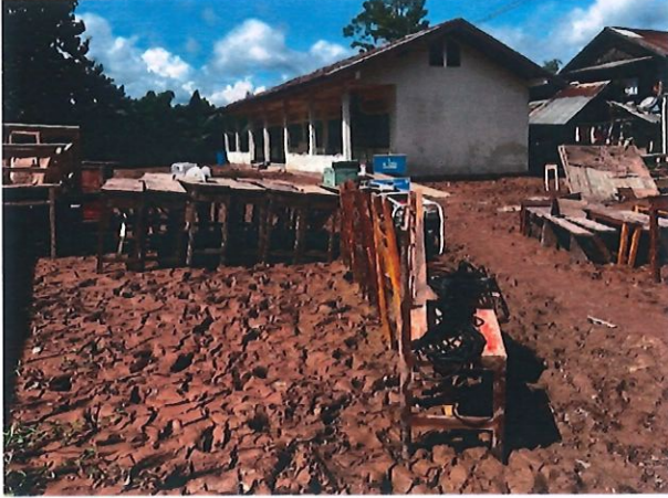
Figure 8: A primary school in Mai Village, Namtha District, is undergoing cleaning and repairs by volunteers
