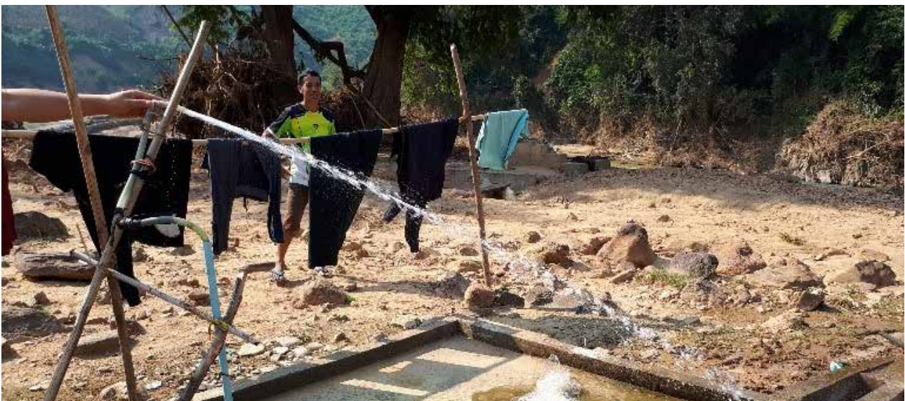
Gravity-fed water supply system damaged by flood in Xiengkhuang Province.
