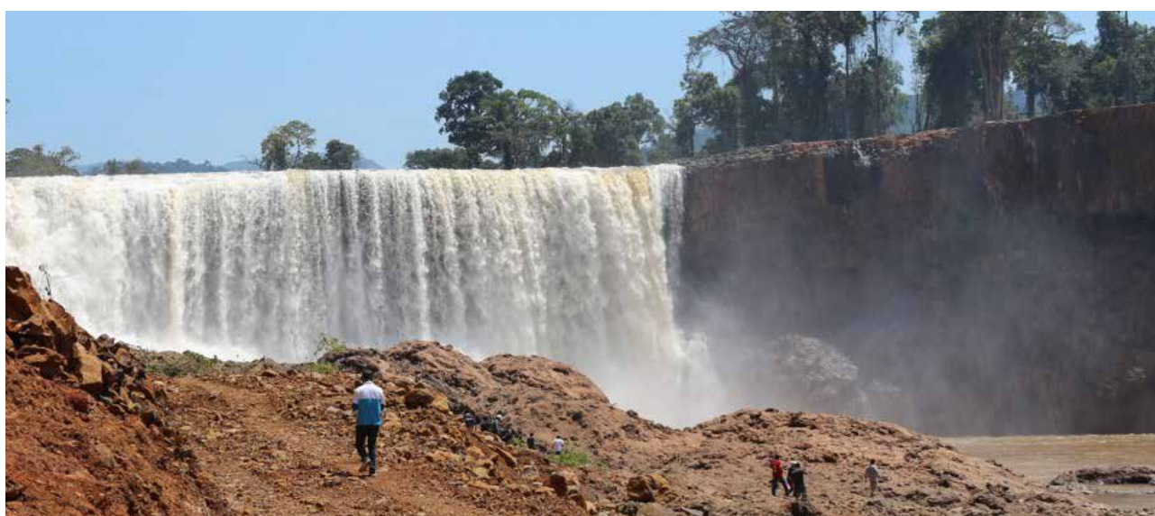
Xe Pong lai Waterfall, showing the damaged area at the base of the waterfall, Sanamxay District, Attapeu Province.
